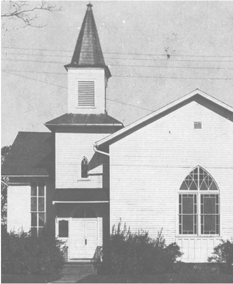
The bell tower was built for our bell in 1911.
